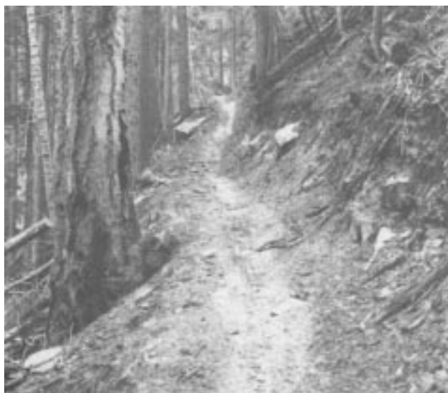
Trees located on the downhill side help to center traffic on the trail.
