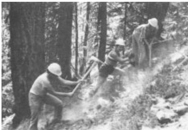
Hand construction is used on More Difficult and Most Difficult trails.
