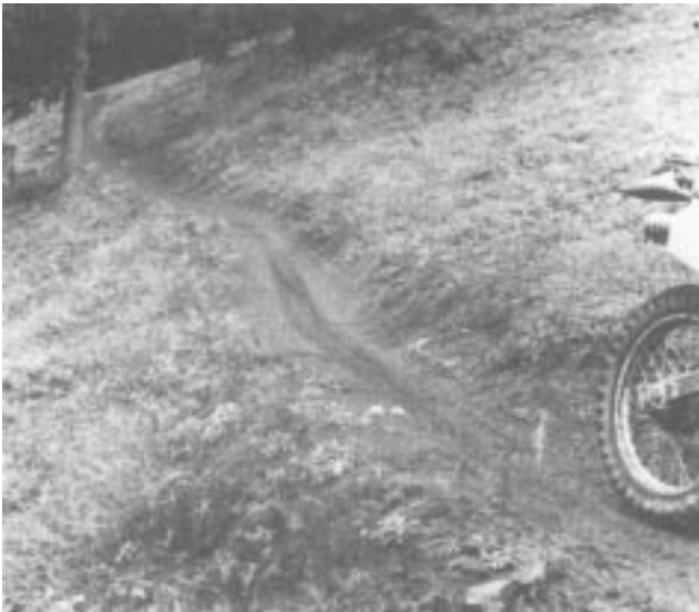
This well-designed trail lays easily on the terrain and creates virtually no adverse impact. There is adequate sideslope to provide drainage away from the trail surface.
