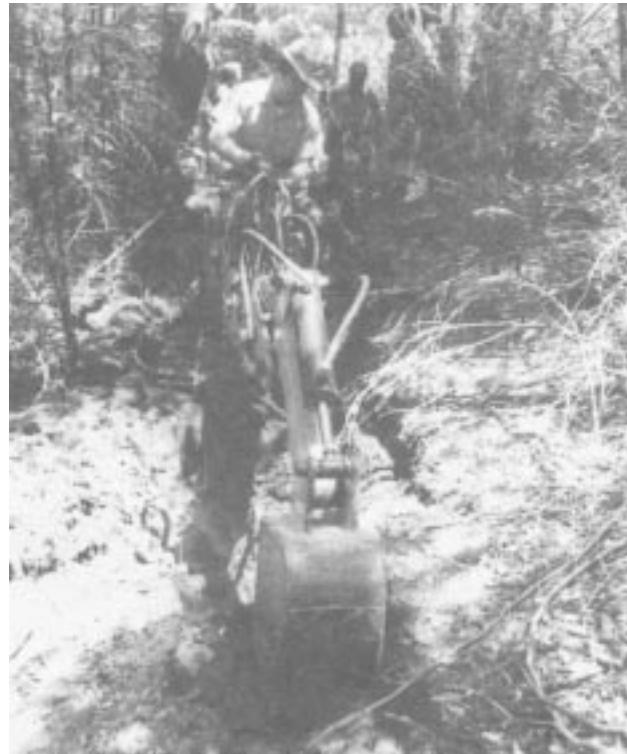
The Morrison Trail Blazer and other similar machines are effective trail building tools.
