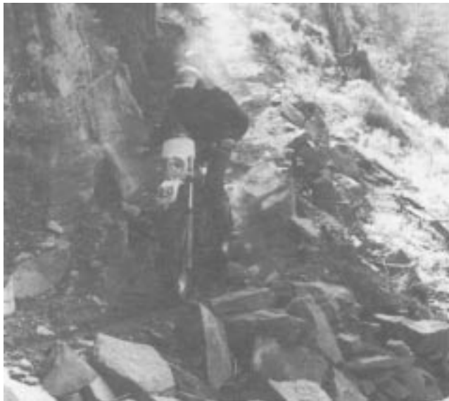
Rock outcroppings often require blasting to build a trail.
