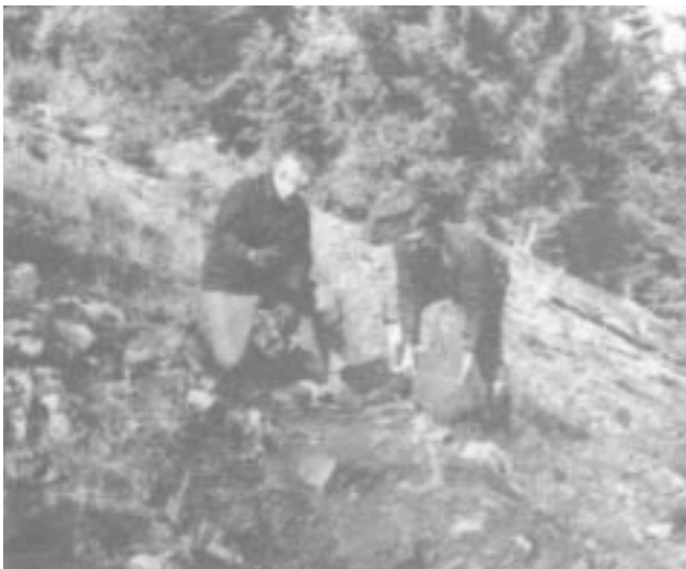
Here, volunteers maintain a section of trail by clearing rocks and other material from the trail tread.
