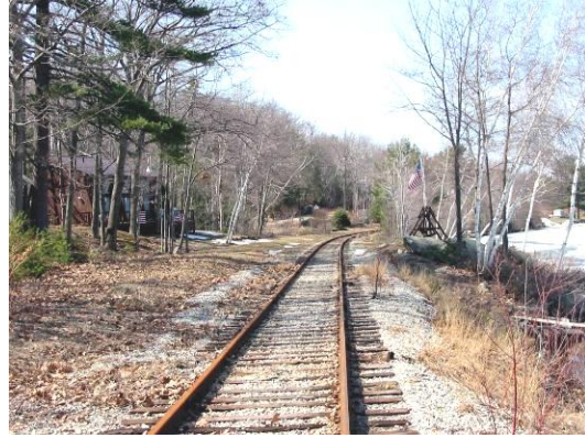
The path would continue on the west side of the railroad, offset from the tracks by about 24 feet in most locations.
