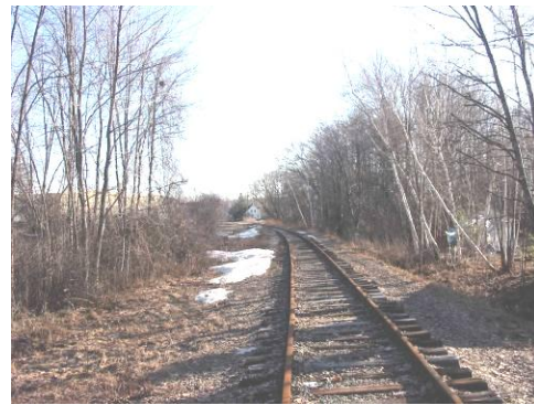
Looking north from Bartlett Beach crossing
