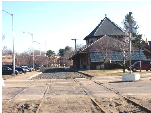
Pleasant Street grade crossing, looking north at Laconia Station
