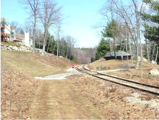
North of the dirt road crossing, the trail would be supported by a low retaining wall on the left side of the railroad.
