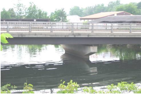
Fair Street Bridge over the Winnepesaukee River
