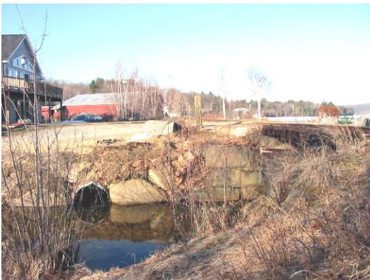
Site of timber trail bridge over Durkee Brook (looking south)
