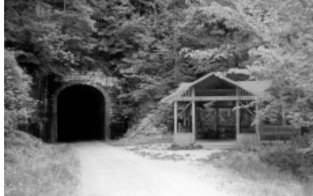
Tunnel #13 along the North Bend Trail in West Virginia. Mark Twain referred to the original railroad corridor as the "Appalachian Subway." Credit: West Virginia State Parks.
