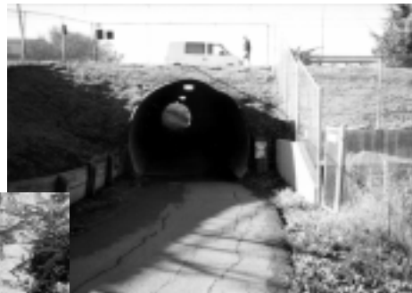
An example of a corrugated metal drain pipe tunnel can be found along the Contra Costa Canal Trail in Concord, Calif. Credit: East Bay Regional Park District.
