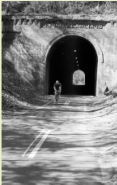
The Dalecarlia Tunnel along the Capital Crescent Trail. Credit: Coalition for the Capital Crescent Trail.
