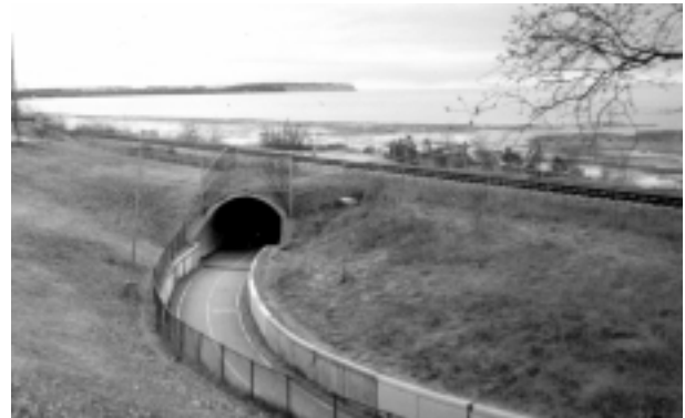
This is an example of a “cut and cover” tunnel. Tony Knowles Coastal Bike Trail, 10 Anchorage, Alaska. Opened 1987. Credit: Jack Mosby.
