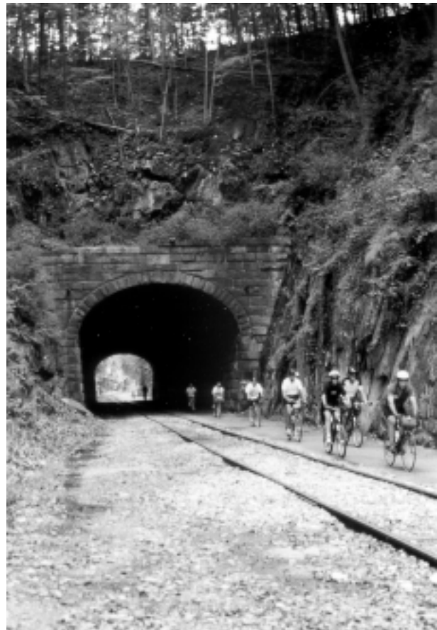
Howard Tunnel, York County Heritage Trail, Penn. This is the only rail-with-trail tunnel that was identified for this report. Tourist trains must wait for tunnel users to exit the tunnel before proceeding. Credit: York County Parks.
