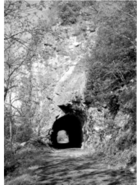
The Austinville Tunnel along the New River State Trail in Virginia is an example of a “mined” tunnel. Credit: Virginia State Parks.
