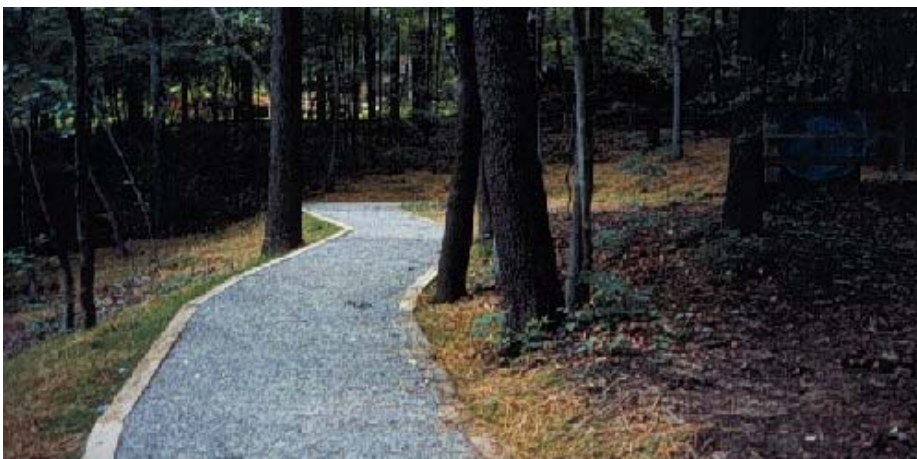
Trail surface with compacted gravel and crusher fines.
