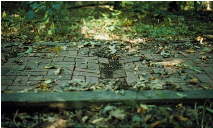
(Left) Brick surface buckled by freezing and thawing. (Right) Asphalt surface edge breaking away.
