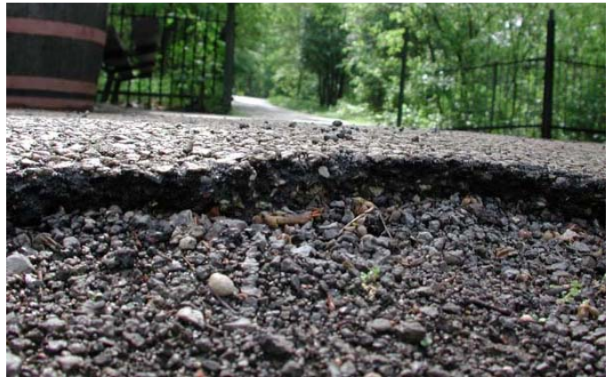
(Left) Brick surface buckled by freezing and thawing. (Right) Asphalt surface edge breaking away.
