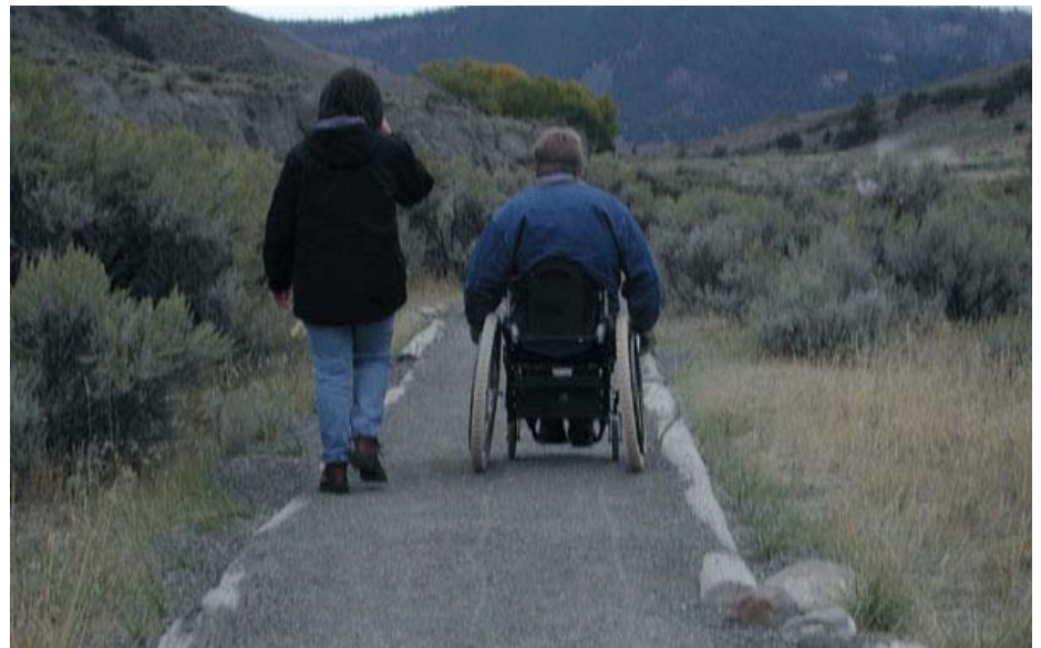
Crushed fine surface used on the Boiling River Trail at Yellowstone NP.
