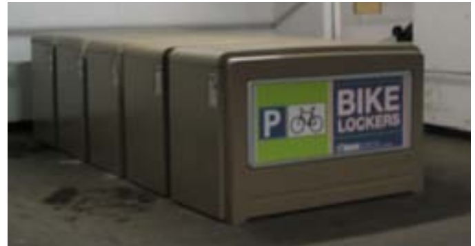
Bicycle lockers in an underground parking garage (Ontario Institute for Studies in Education, University of Toronto).
