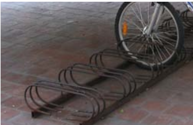
This "wheel bender" rack does not allow bicycle frames to be securely locked to the rack.
