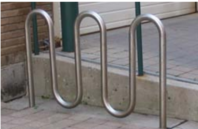
Bikes park at 90° angles to this rack which only provides 1 point of contact per bike. If installed too close to an obstacle, like this rack, capacity is reduced to 1 or 2 bikes at most.
