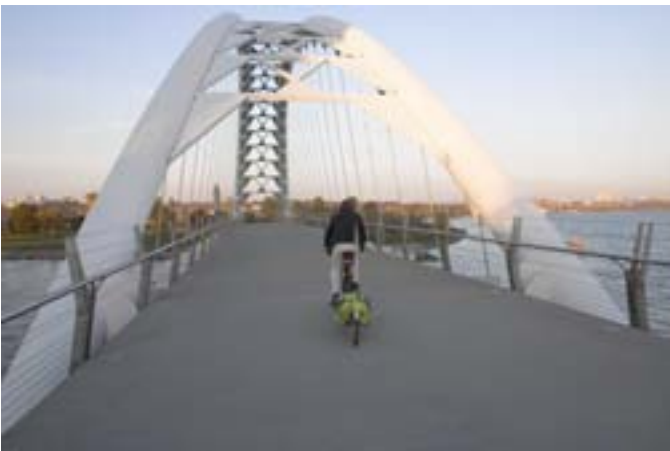
Humber river pedestrian and bicycle bridge
