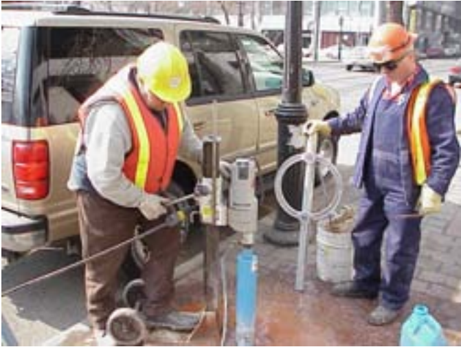
City of Toronto staff installing post-and-ring bicycle parking in the public right-of-way.
