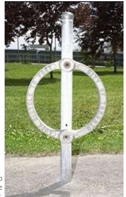
City of Toronto Post-and-Ring bicycle parking rack.
