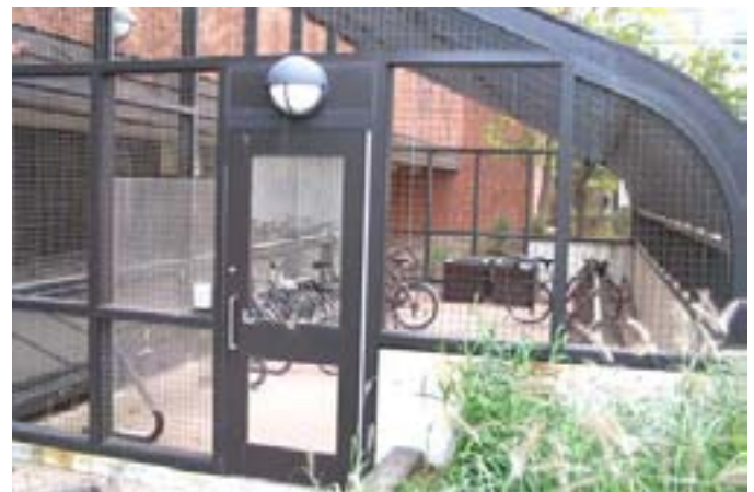
Bicycle cage at Toronto Reference Library (Glass roof extends down from main building, wire mesh walls, restricted access through electronic key pad).
