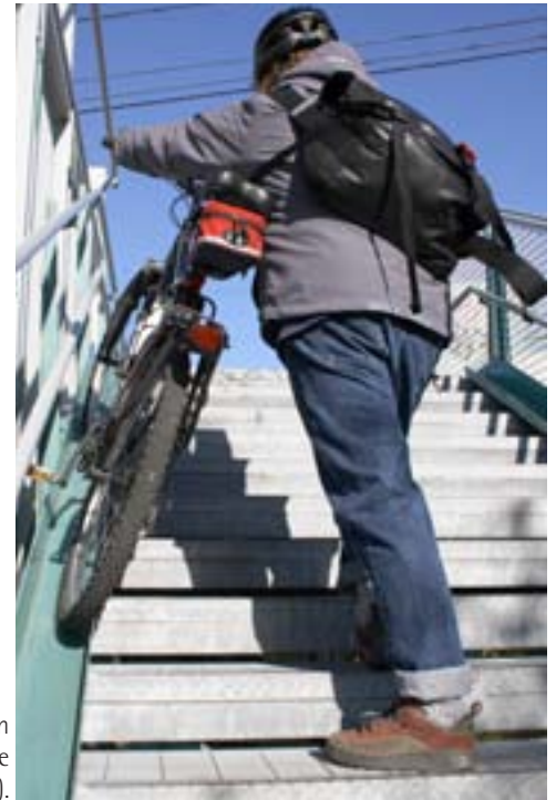
Bicycle ramps on stairway (Riverdale Park, Toronto).
