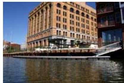
Buffalo Street Access (Photo: FMR)
