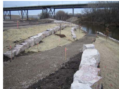
Access open in 2006 (Photo: MVP)
