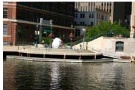
Mason Street Access (Photo: FMR)
