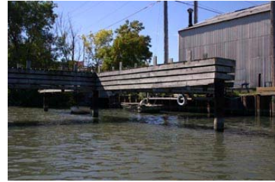
Pier along shoreline behind fixed pier (Photo: FMR)
