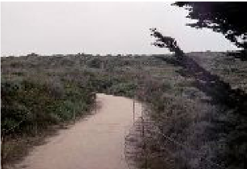
Many trail managers are beginning to utilize non-petroleum based surfacing -- hardness and cost are similar to asphalt.
