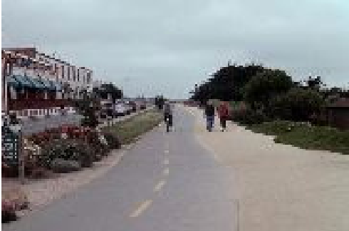
Recommended design for multi-use trails with paving include an unpaved shoulder for those who don't want a paved surface.
