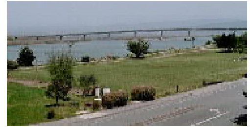
A study of alternatives for redevelopment of the Carson Mill Site was recently completed.
