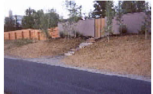
Appropriate fencing can enhance the overall character of a trail corridor.
