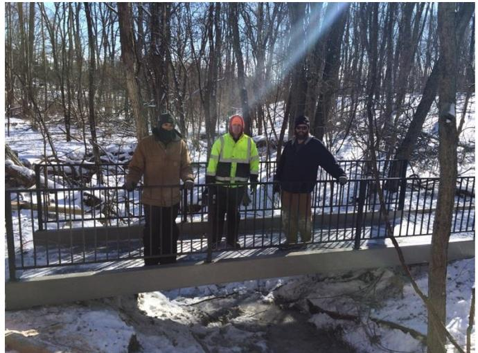
“The anti-slip wearing surface provides excellent slip resistance,” Pion adds. “We expect this surface to perform well in our all-weather trail application.” The fiberglass bridge was delivered to the site with curbs and steel railings attached; and meets the industry standard of 90 pounds per-square-foot pedestrian live load.
